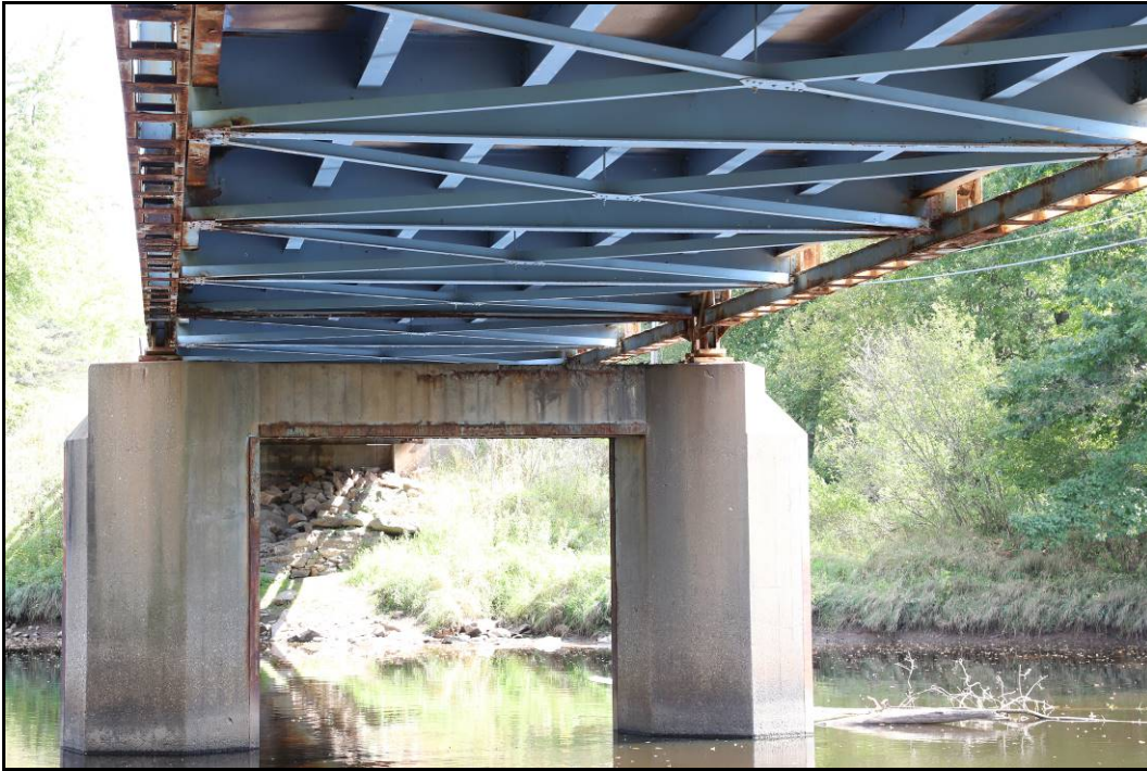
Figure 6: AHI #243375. View to ESE. Pier, deck beams, floor beams and stringers.
